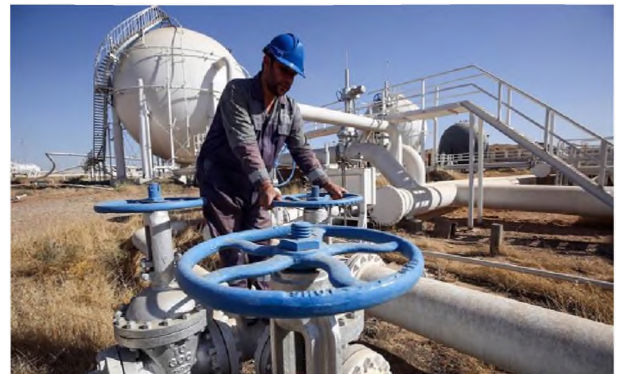
A worker checks pipelines at the Bai Hassan oil field in Kirkuk, October 2017. File photo: Ahmad Al-Rubaye / AFP
