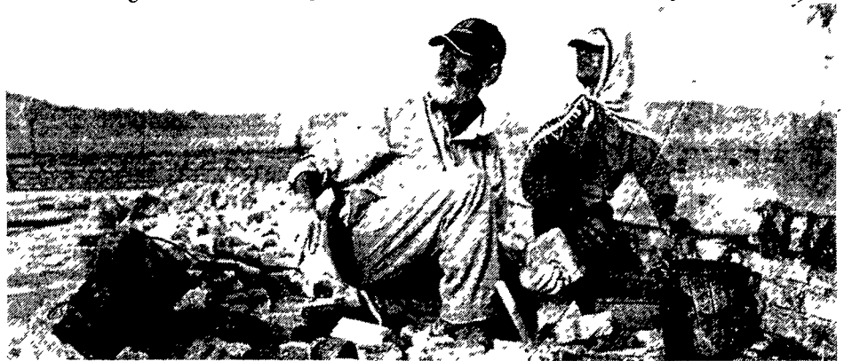
Afghan subcontractors building a school as part of the reconstruction effort in Herat, near a library built by Iran.
