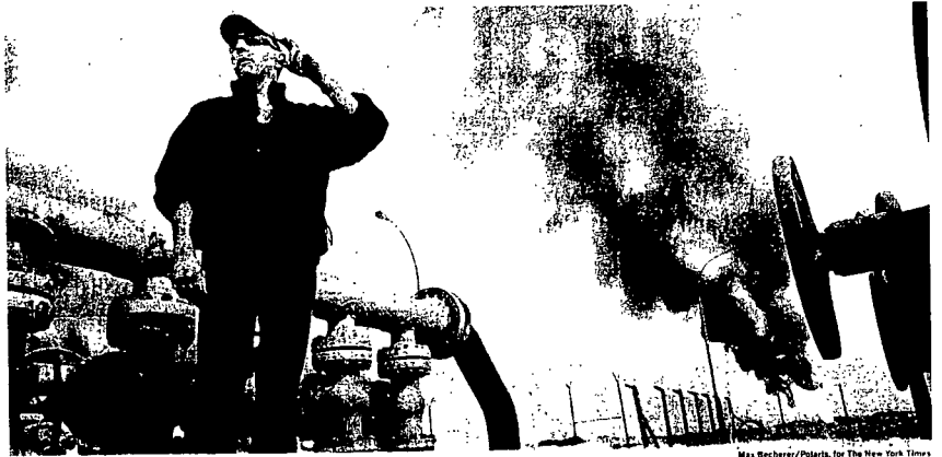
⚙️ Althaus, a manager with Kellogg, Brown & Root, at an Iraqi oil plant where an oil byproduct that could be turned into liquified gas is simply burned off instead.
