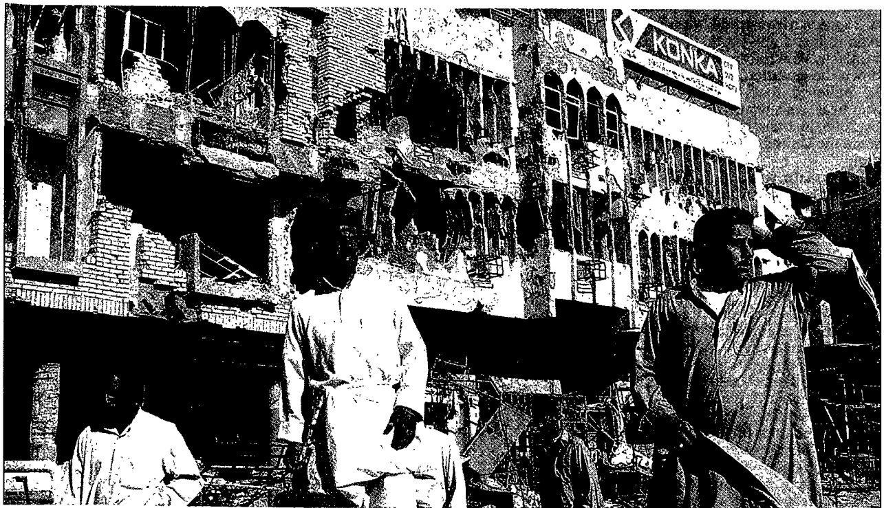
Iraqis survey the damage to the old city in Najaf on Friday near the Imam Ali Shrine after three weeks of fierce fighting.
