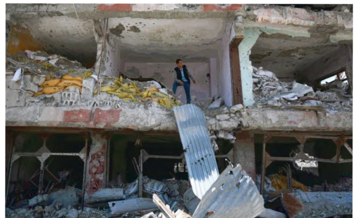
A man stands inside a building which was damaged during security operations and clashes between Turkish security forces and Kurdish militants, in Yuksekova in the southeastern Hakkari province, Turkey, May 30, 2016. REUTERS/Sertac Kayar
