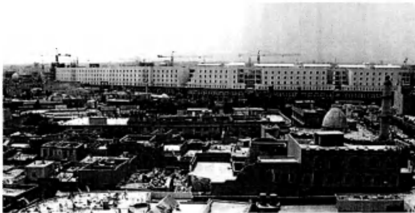
Construction cranes dot the skyline as a new shopping mall rises in Irbil.
